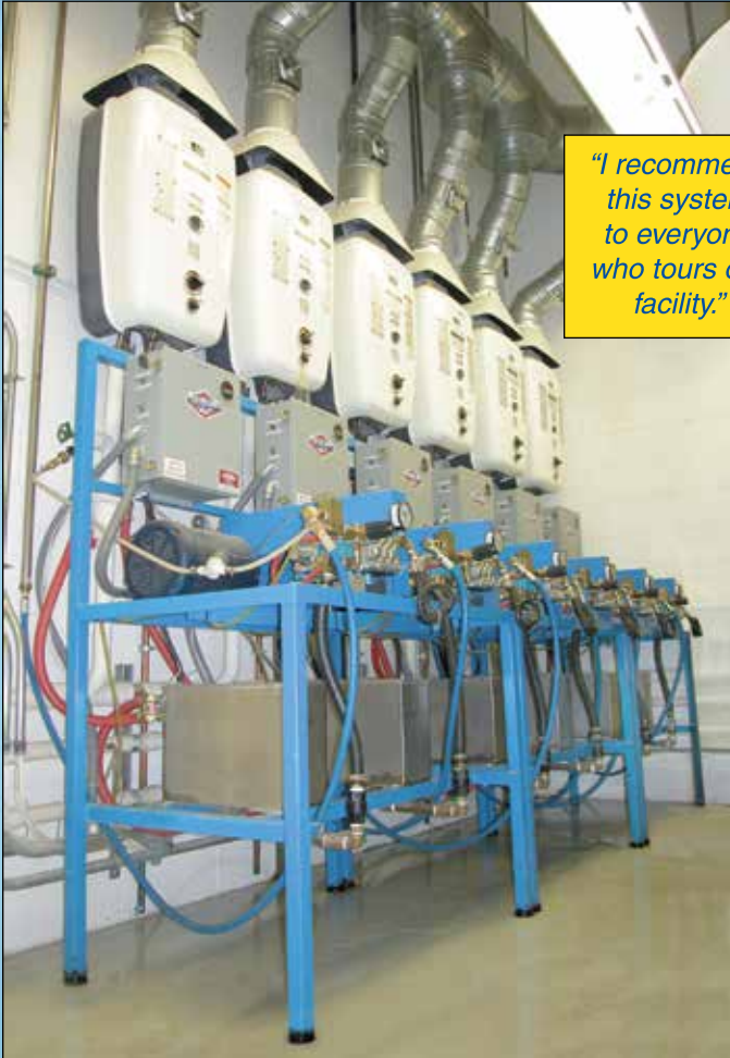
Dultmeier high pressure pump stations inside the Nebraska Humane Society (Omaha, Nebraska) maximize kennel cleaning effectiveness and speed.
